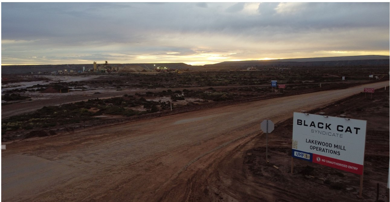
Figure 1: Lakewood processing facility
