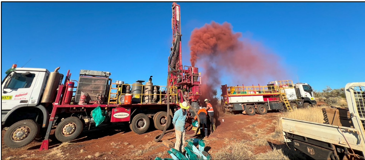
Figure 1: RC drill rig on tenement E46/1407 collaring into the iron formation looking to the east.
