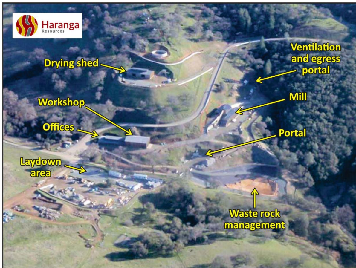
Photo 1: Aerial photo of the Lincoln Gold Mine infrastructure 1 .
