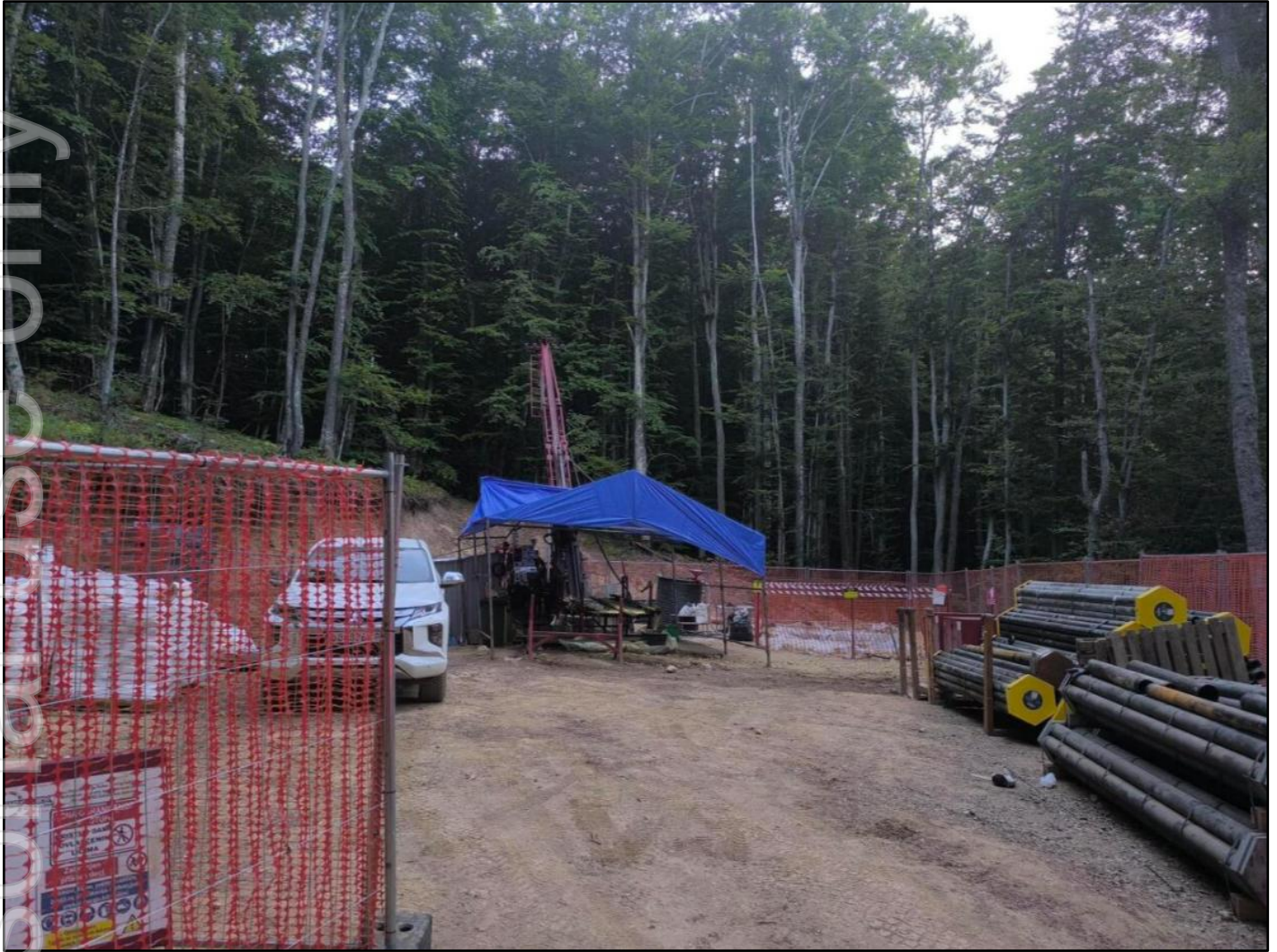
Figure 2. Photo of the eighth diamond rig in action at Shanac.
