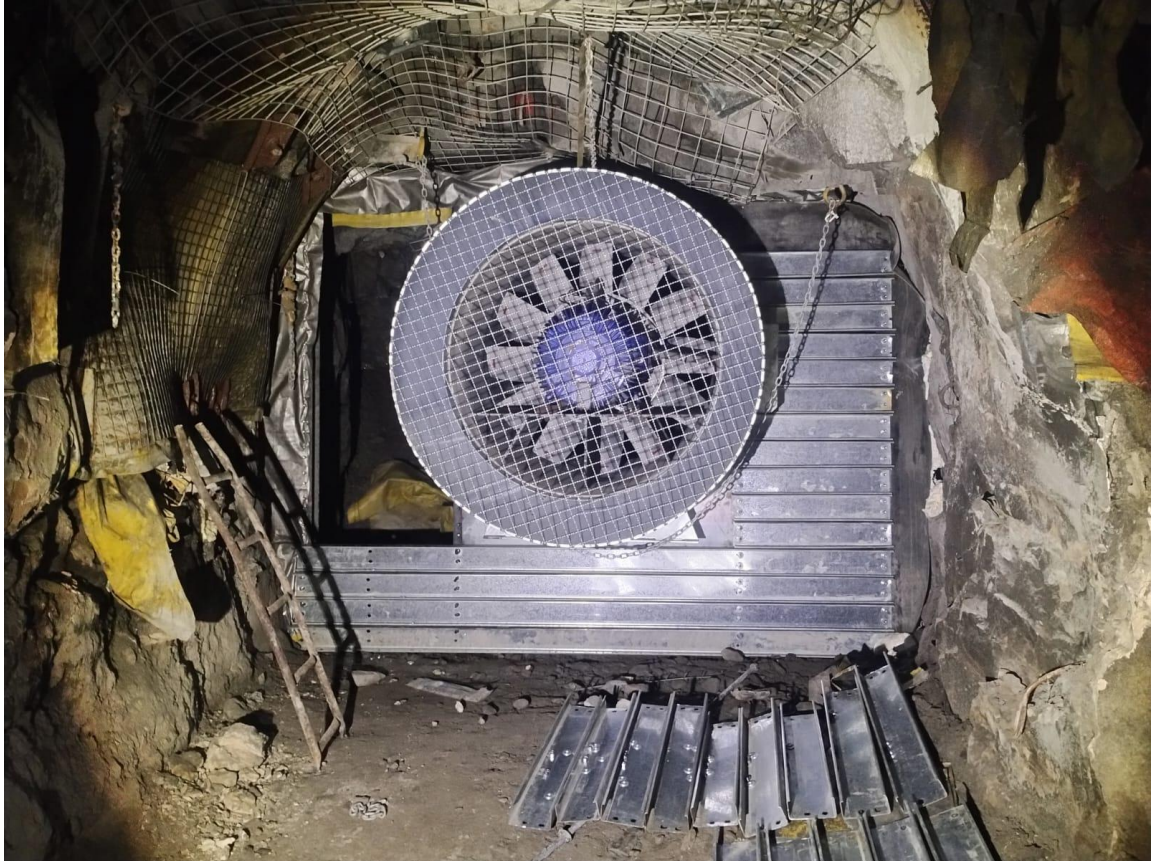
Figure 2 - 110kW primary ventilation fan installed and ready for power
