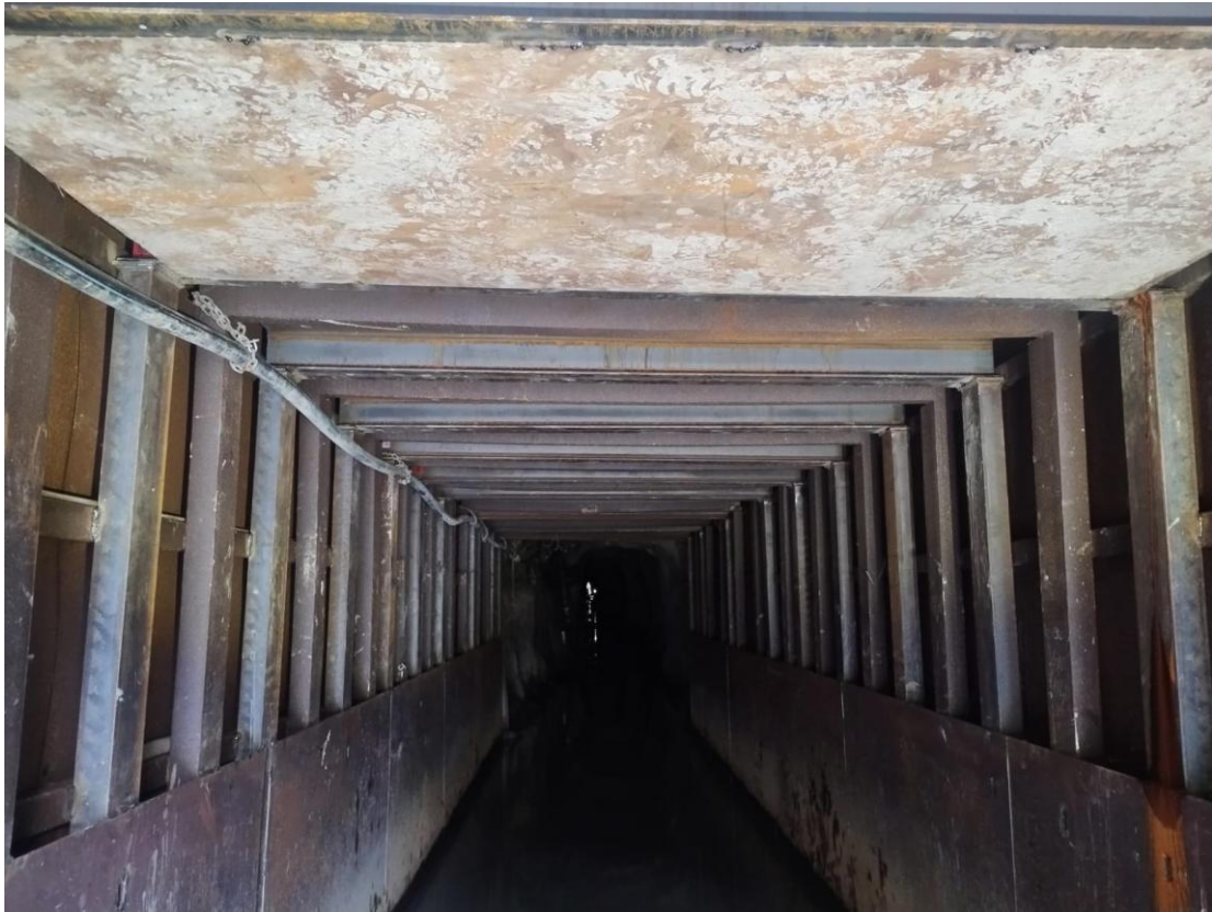
Figure 8 – Upgrade of 25-year-old steel sets at the Amalgamated Portal.
