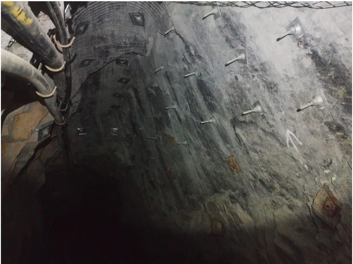
Figure 3 The underground substation caddy completed
