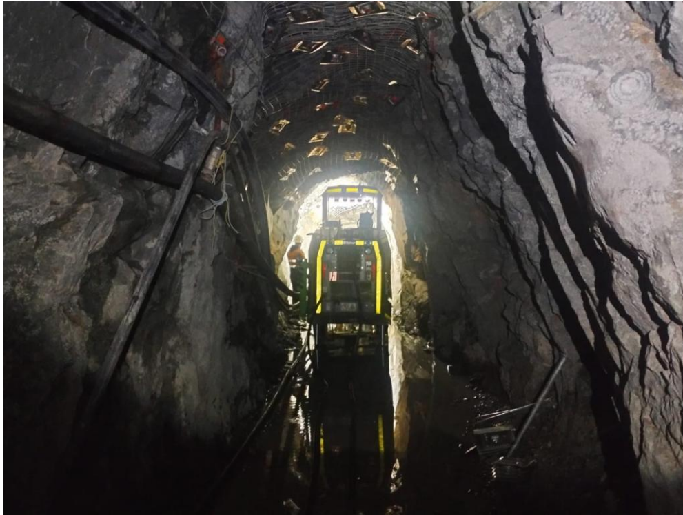
Figure 7. T1D jumbo operational and bolting the main access.
