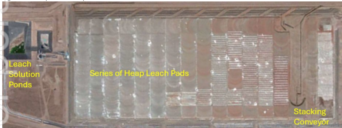
Figure 12 - Sequential Heap Leach Pads
