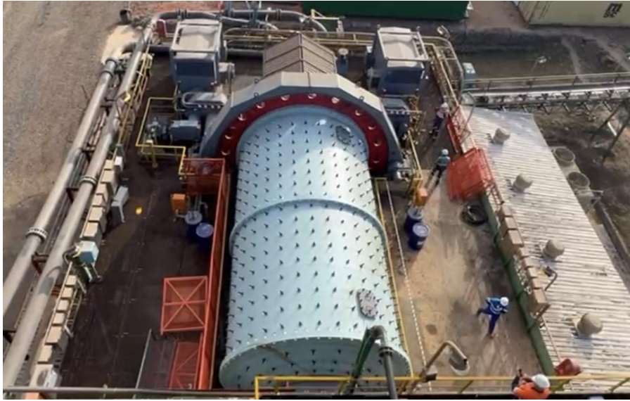
Figure 1: SAG mill refurbishment completed
