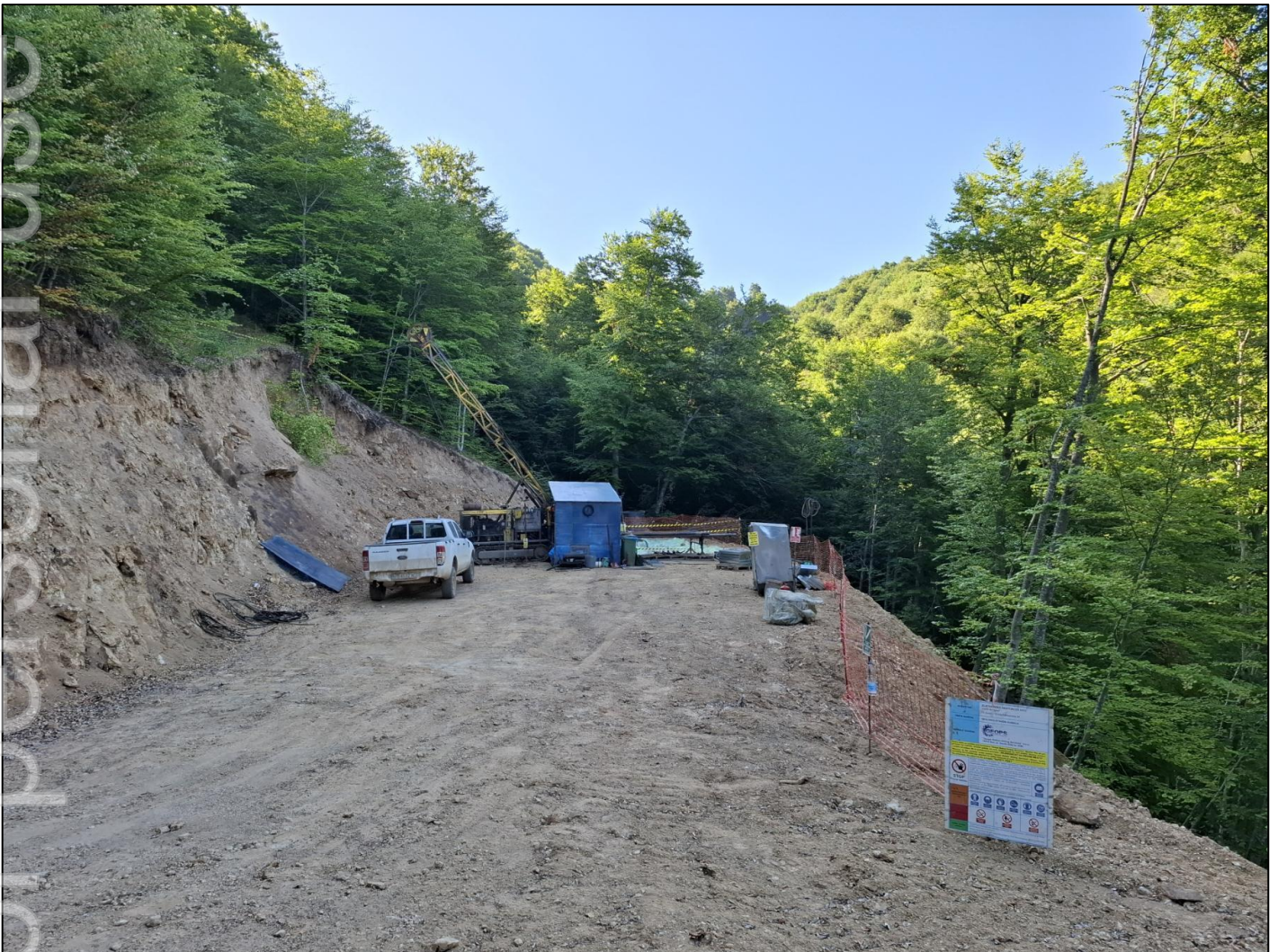
Figure 2. Photo of the drill rig operating at Jezerska Reka.
