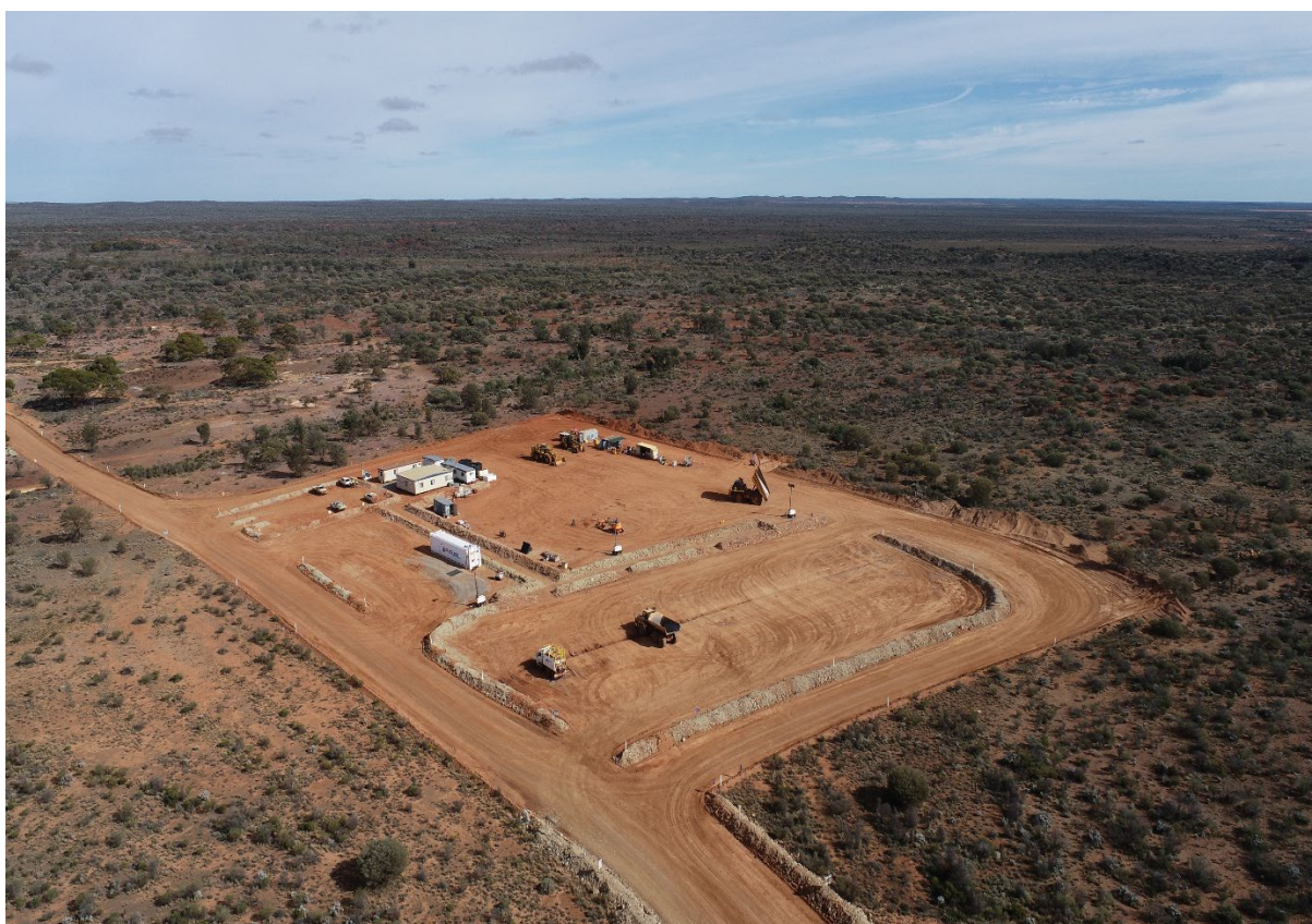
Plates 8 & 9 Mine offices, workshop and medical centre under construction (May 2025)
