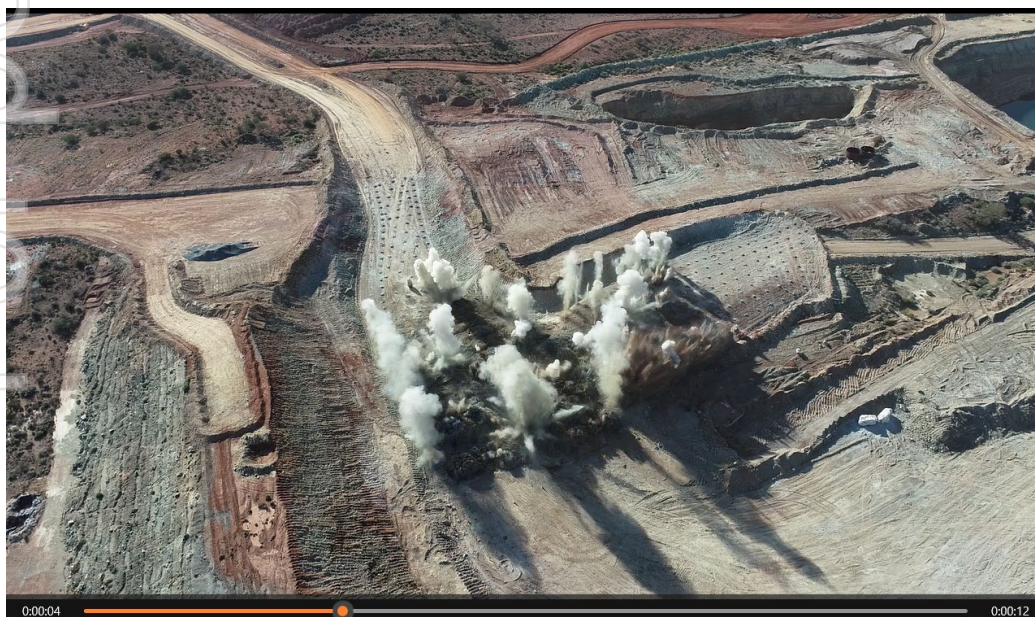
Stage 1 West Lode blast 10 July 2025 (drone view looking east)
