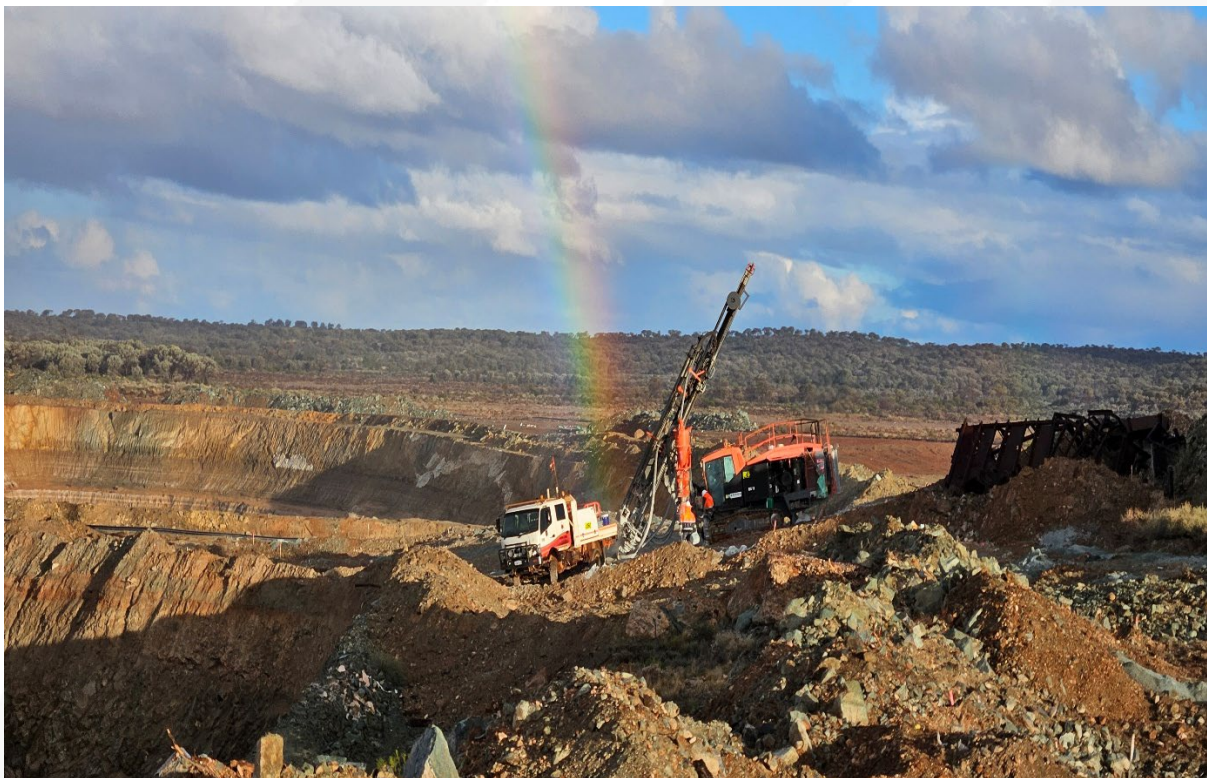
Plate 1 – Grade control drilling at Devon (June 2025)
