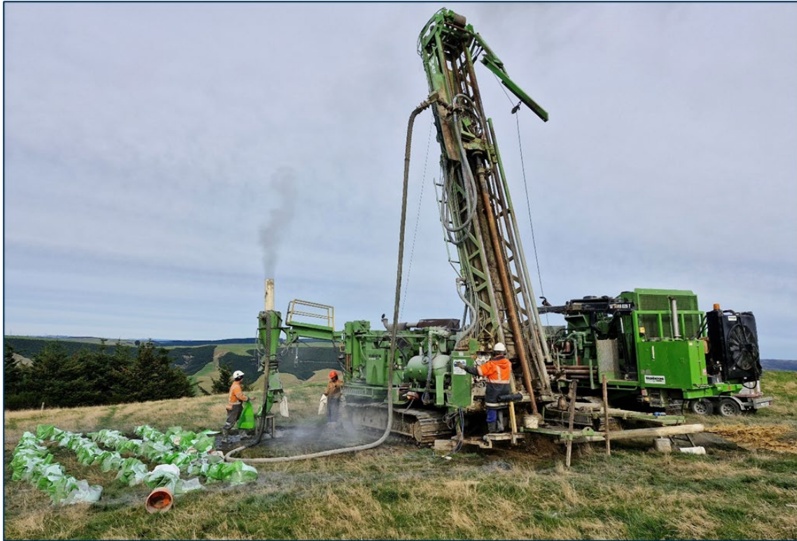
Figure 11: Photo of RC drilling operation on Waipori Station (EP60807 - Lammerlaw)
