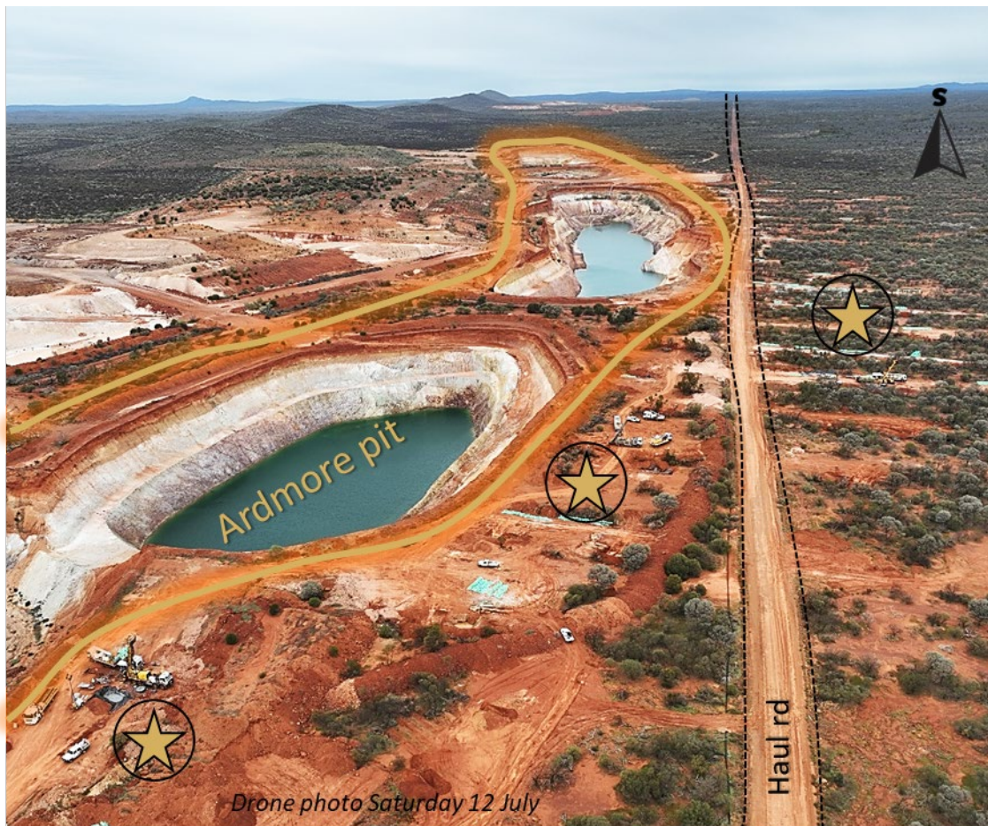
Figure 8: Drone photo (12 July) showing ongoing RC and diamond drilling at Ricciardo. View looking South down the haul road. Stars indicate the location of rigs (the RC rig on the right is a little hard to see).
