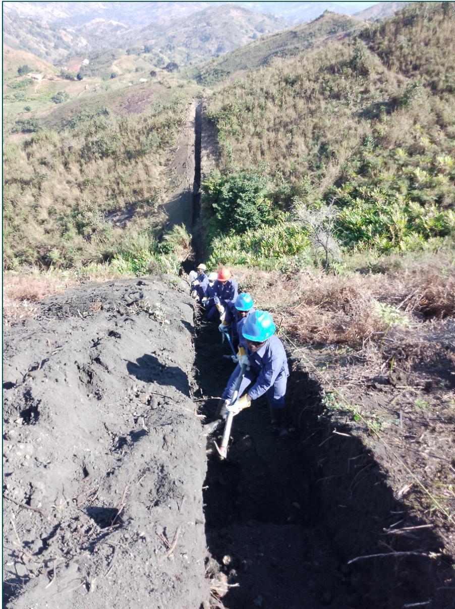
Photo 1: Excavation of trench TRUM23-002.
