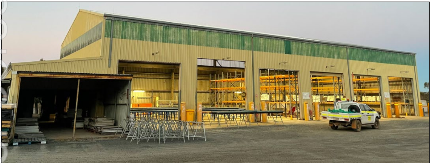
Figure 20: Foster Mine workshop
