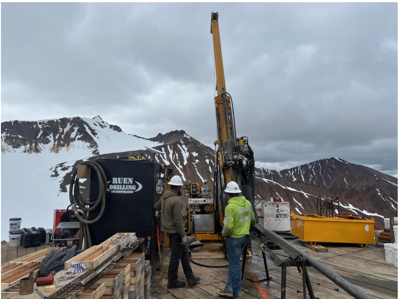
Figure 1. Drilling well underway at RPM North
