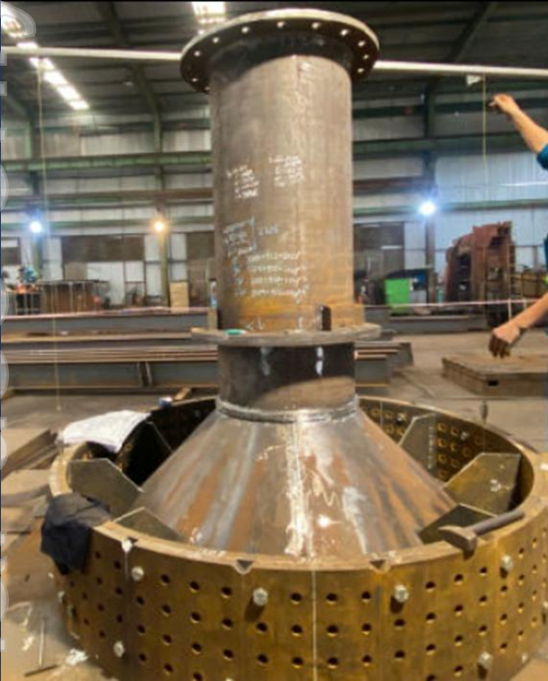
Photo: Thickener in construction in Vietnam
