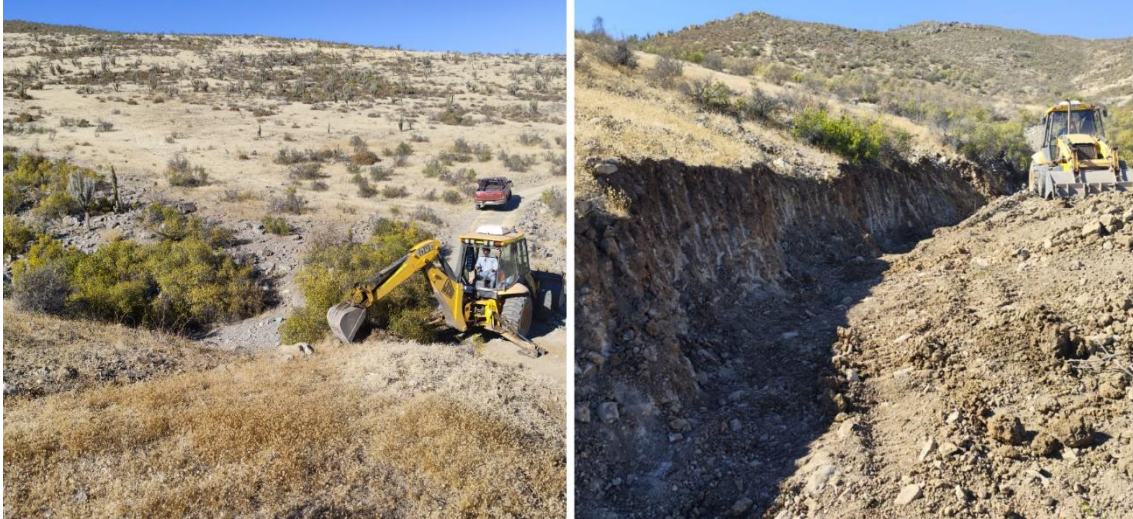
Figure 3: Backhoe working on trench FL013.
