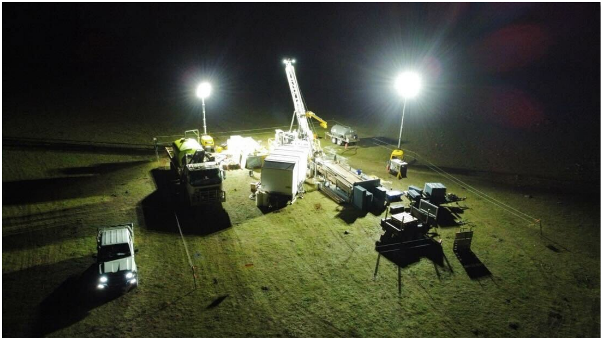
Figure 2. Earth AI drilling onsite at Fontenoy.
