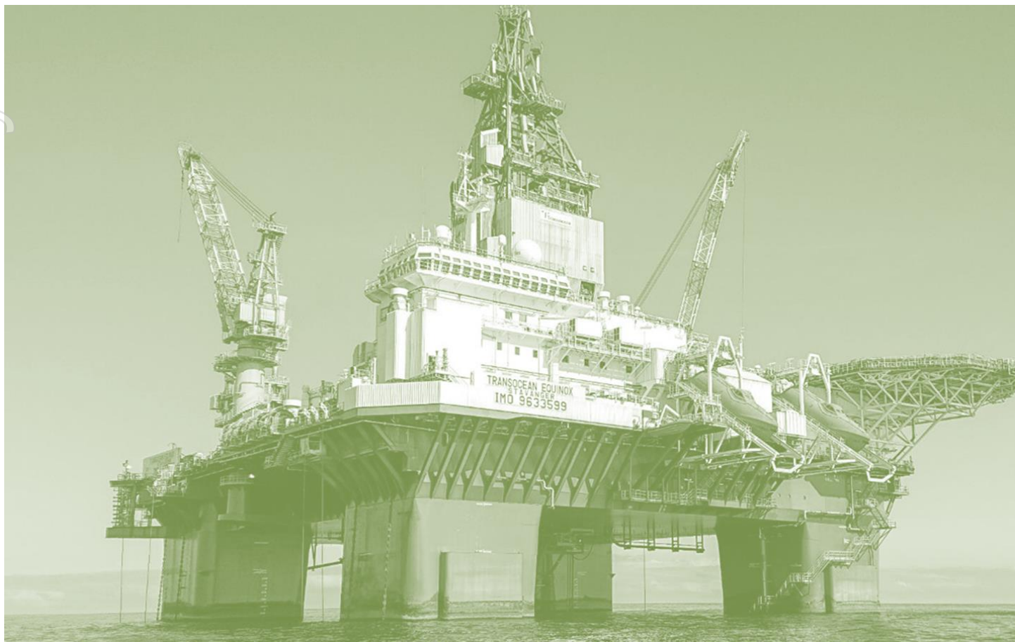
Figure 1: Transocean Equinox semi-submersible drilling rig
