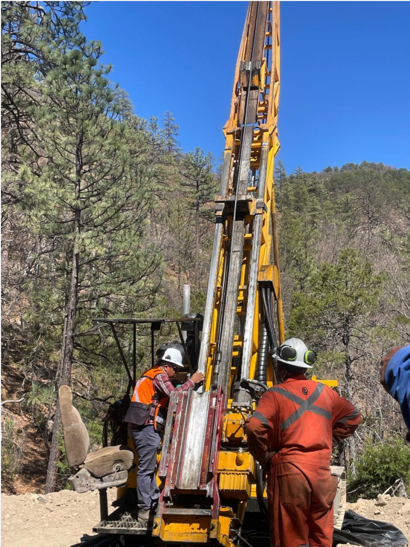
Figure: Photograph of the drilling rig setting up to commence YQ-25-003 in May 2025
