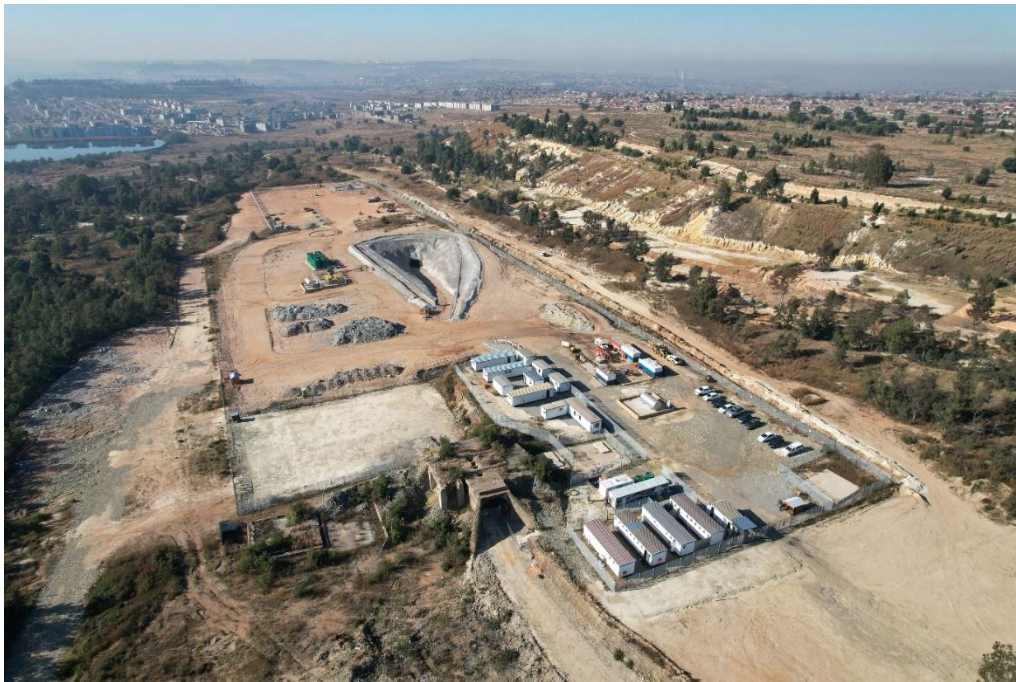
IMAGE 2: QALA SHALLOWS PROJECT PROGRESS
