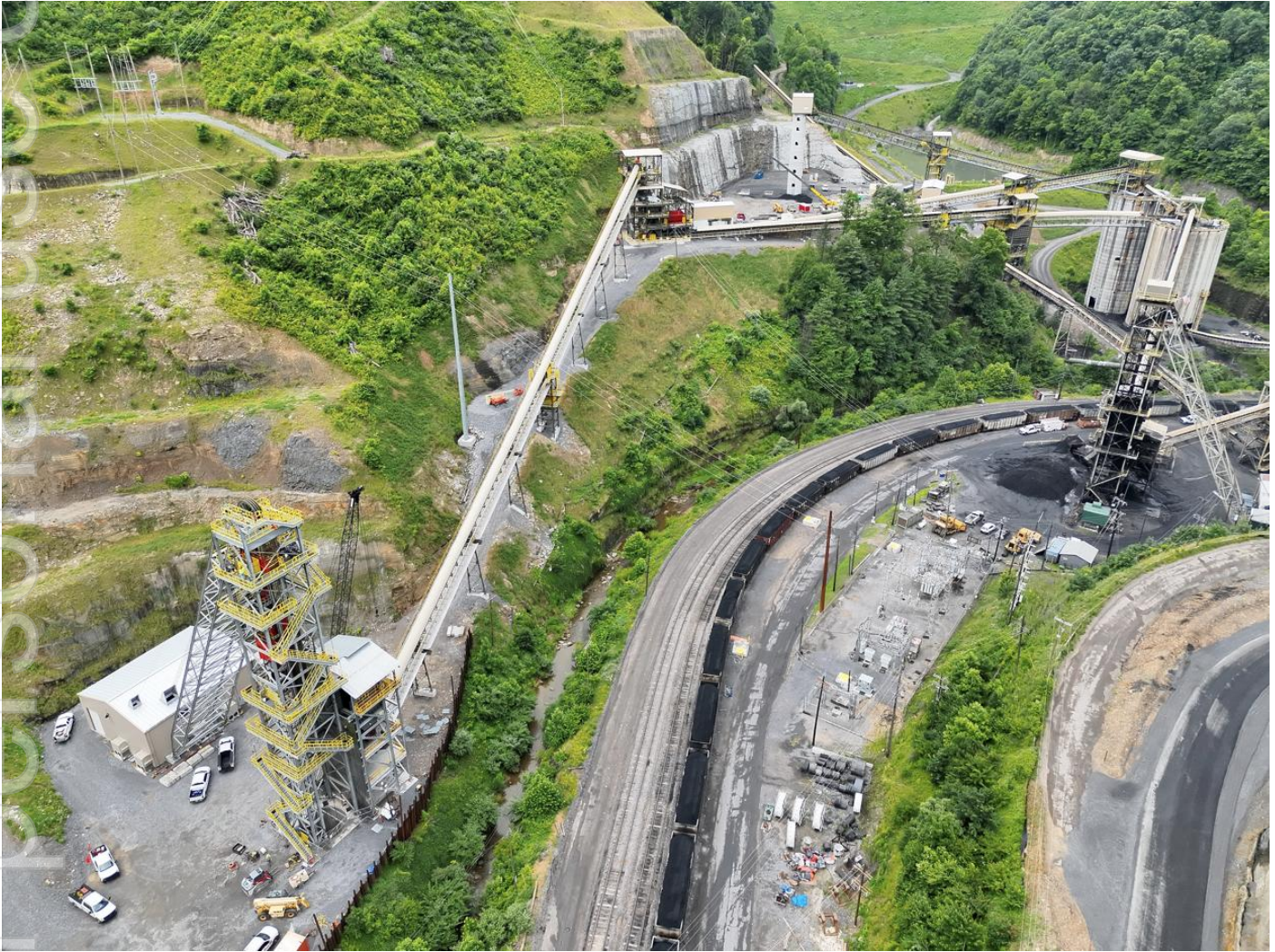
Caption: New Surface Raw Coal Storage Area – Complete
