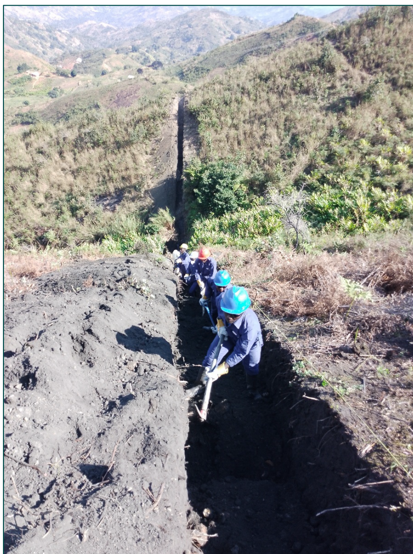
Photo 1: Excavation of trench TRUM23-002
