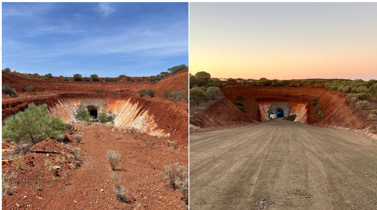
Figure 8: Refurbishment of K2 boxcut and portal
