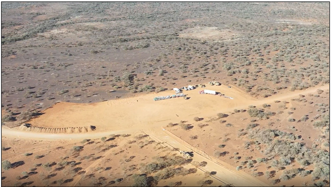
Figure 7: Trident early works – earthworks commencing for offices and workshops
