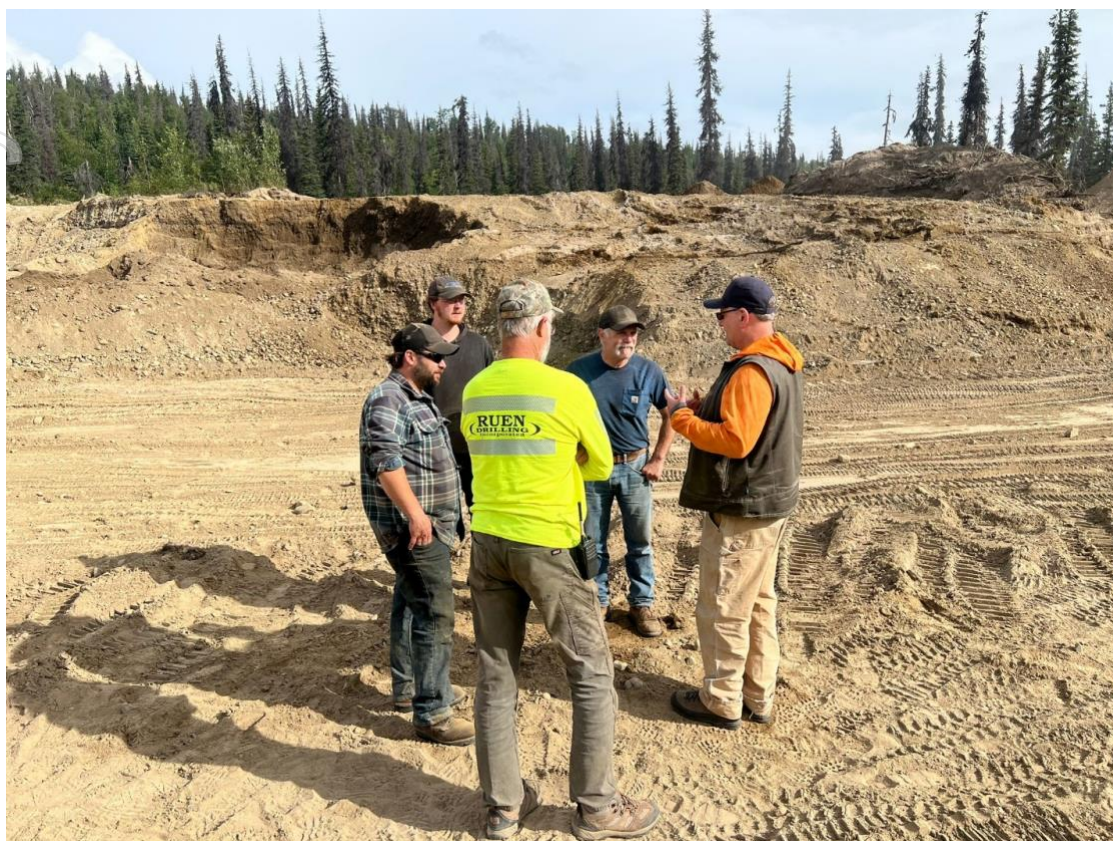
Nova Minerals Directors and CEO, Christopher Gerteisen allocating earthworks within the Estelle project area.
