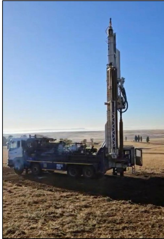
Figure 1: Drilling rig on site for spudding well 271-KA03PT10
