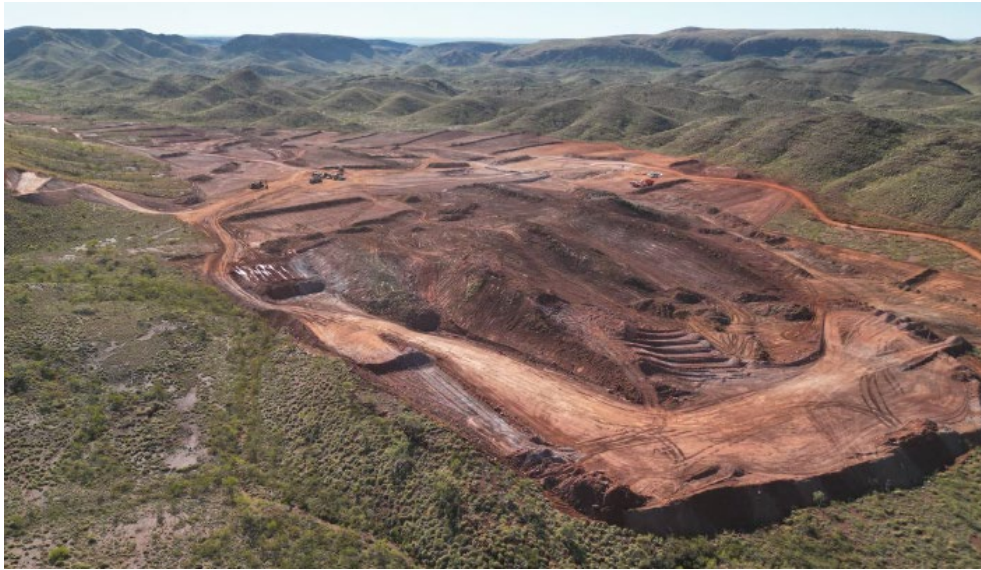
Figure 7: Clearing of the boxcut, mine infrastructure and process plant footprint.
