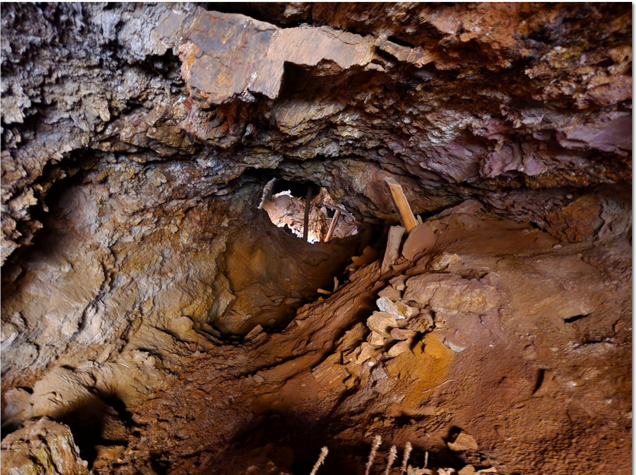
Picture 2a and 2b: Underground Historic Workings at Sunday. The drives are approx 2m x 2m in section, and the shafts range in depth from 7m to 25m .
