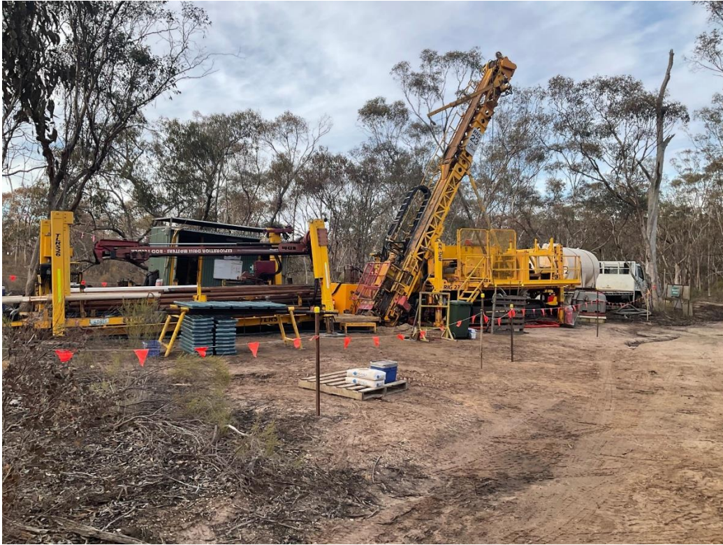
Figure 2. Drilling at Crosbie South
