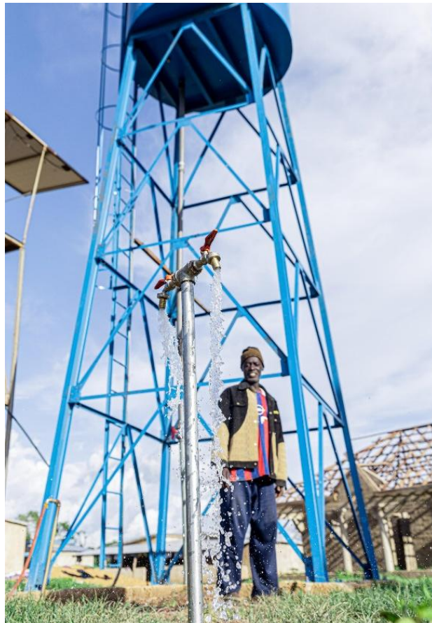
Figure 5: Toubani sponsored the installation of a new water tower for the Faraba village
