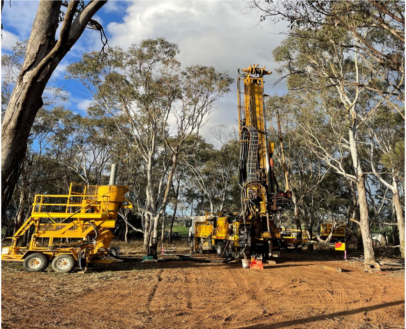
Figure 1: Drill Rig mobilised at Gidginbung gold deposit
