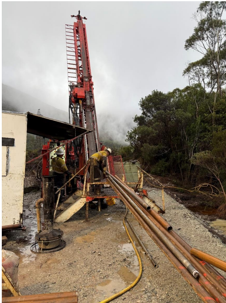
Figure 2 – Drill rig at Tyndall Creek, 29 April 2025
