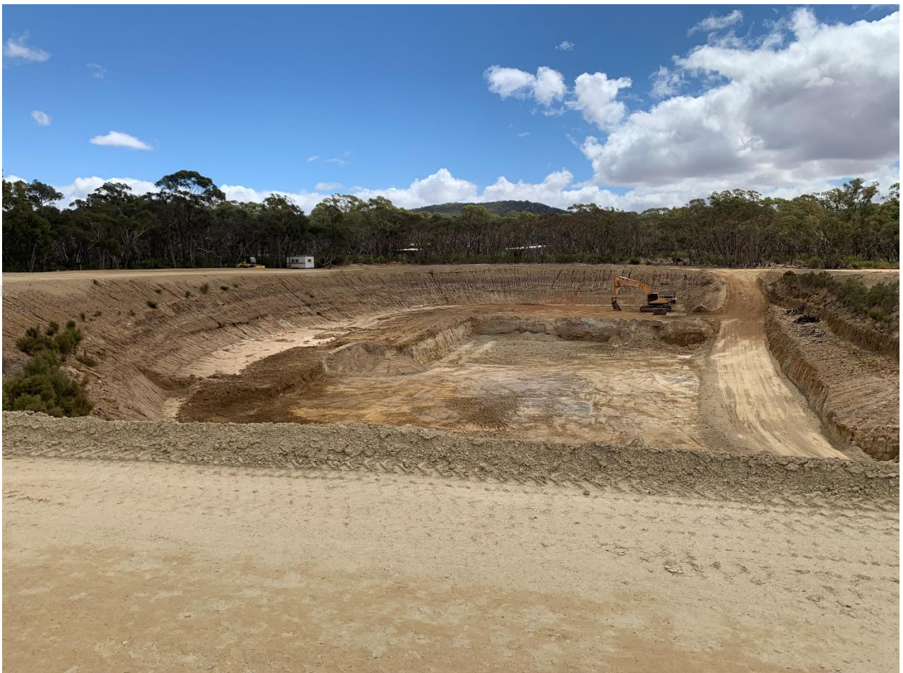
Figure 8 – Tails dam lift nearing completion, incorporating existing borrow pit area
