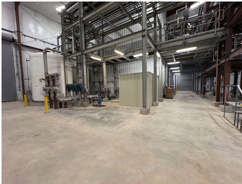
Inside the CPP Phase 2
