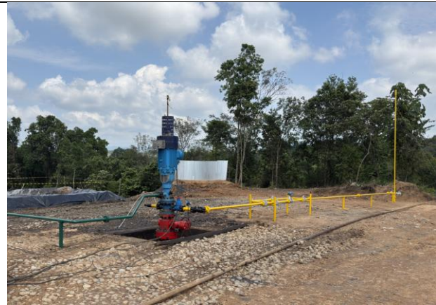
Dewatering Activity Well TE B06-001
