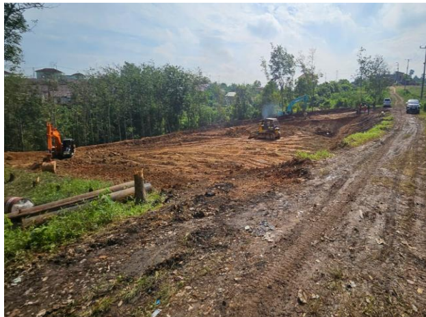
Drill Site Preparation on TEB01003
