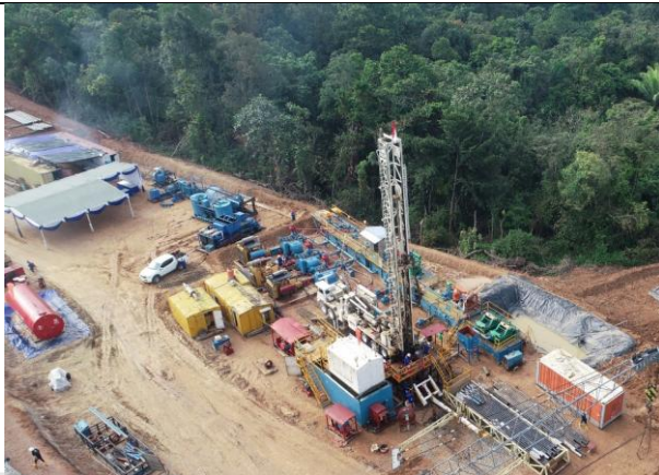
Drilling Activity Well TE B06-001
