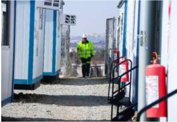
Office infrastructure equipped with modular units, safety signage and firefighting equipment
