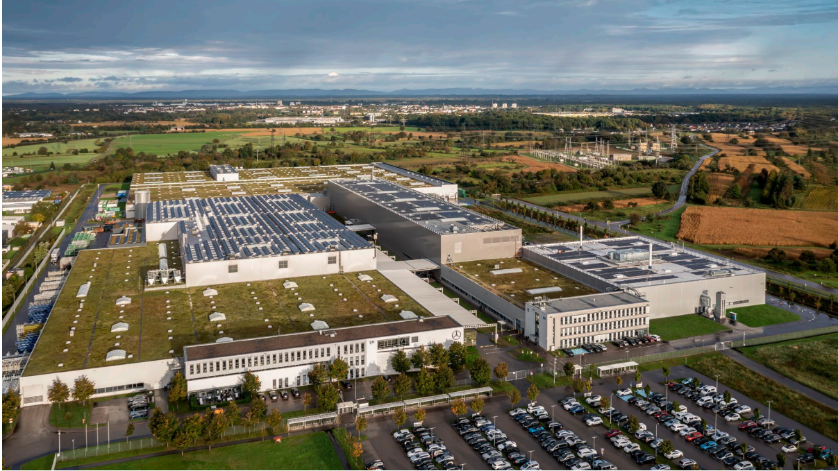
Figure 5 – Recycling Plant Building (far right) at Mercedes-Benz, Kuppenheim
