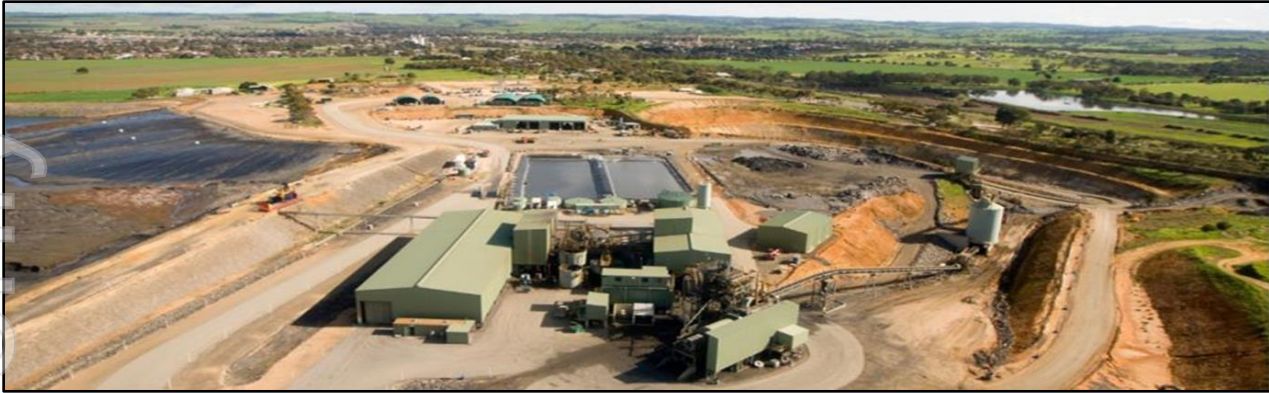
Figure 2: Angas Mine (100% TZN) Existing Processing Plant
