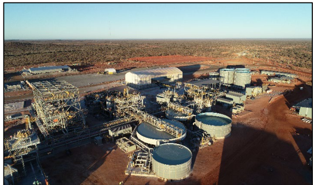
Figure 7: Aerial view of thickener and process water tanks
