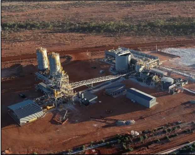
Figure 4: 4Mtpa capacity Paste Plant
