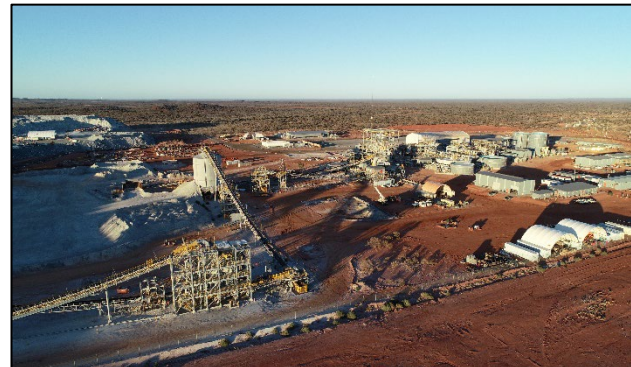
Figure 9: Aerial view of crusher circuit, fine ore bin and plant
