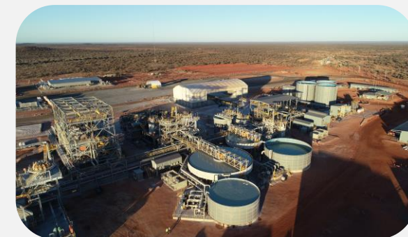
Aerial view of plant
