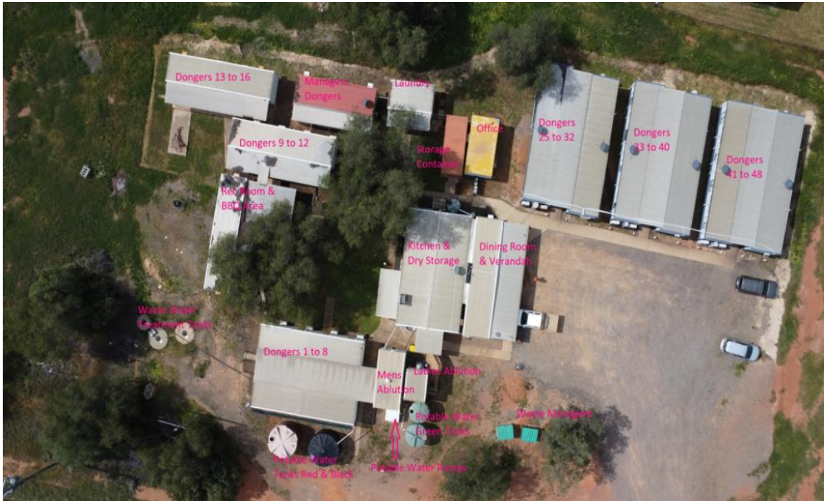
Figure 8: Existing camp facilities located at Mt Boppy
