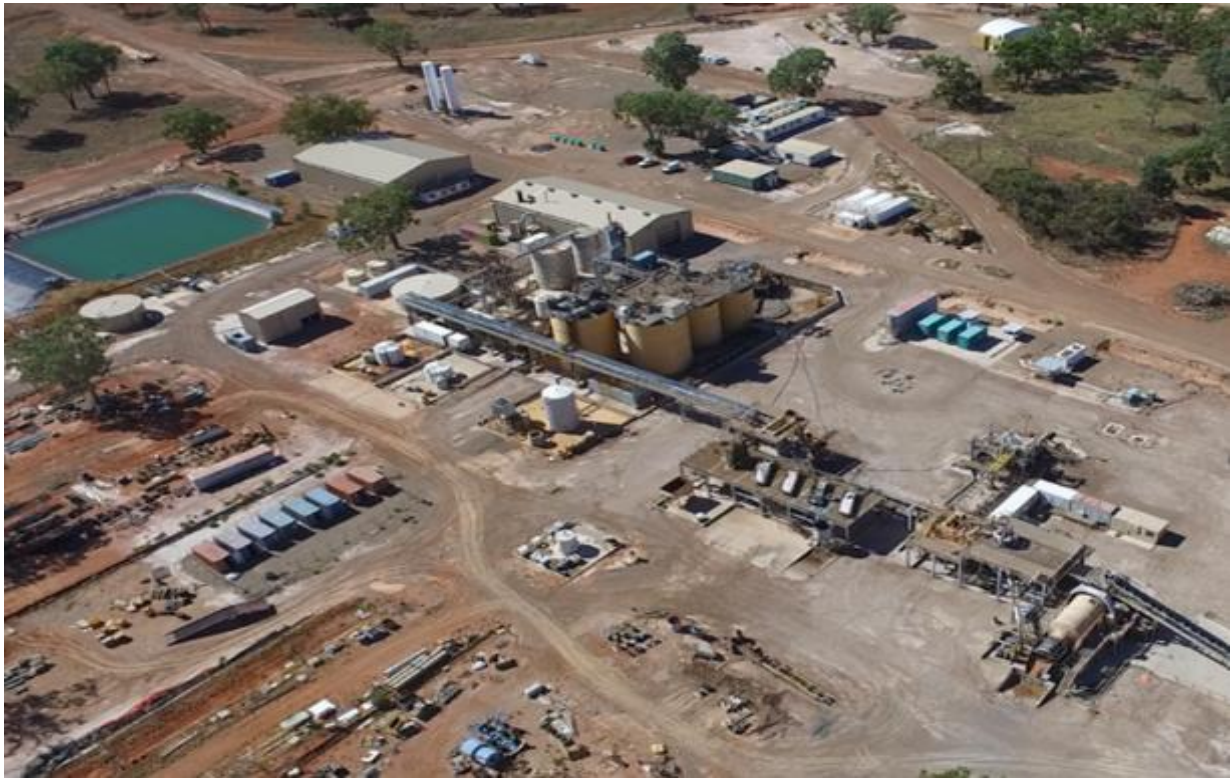
Figure 3: The existing Wonawinta Processing Plant.
