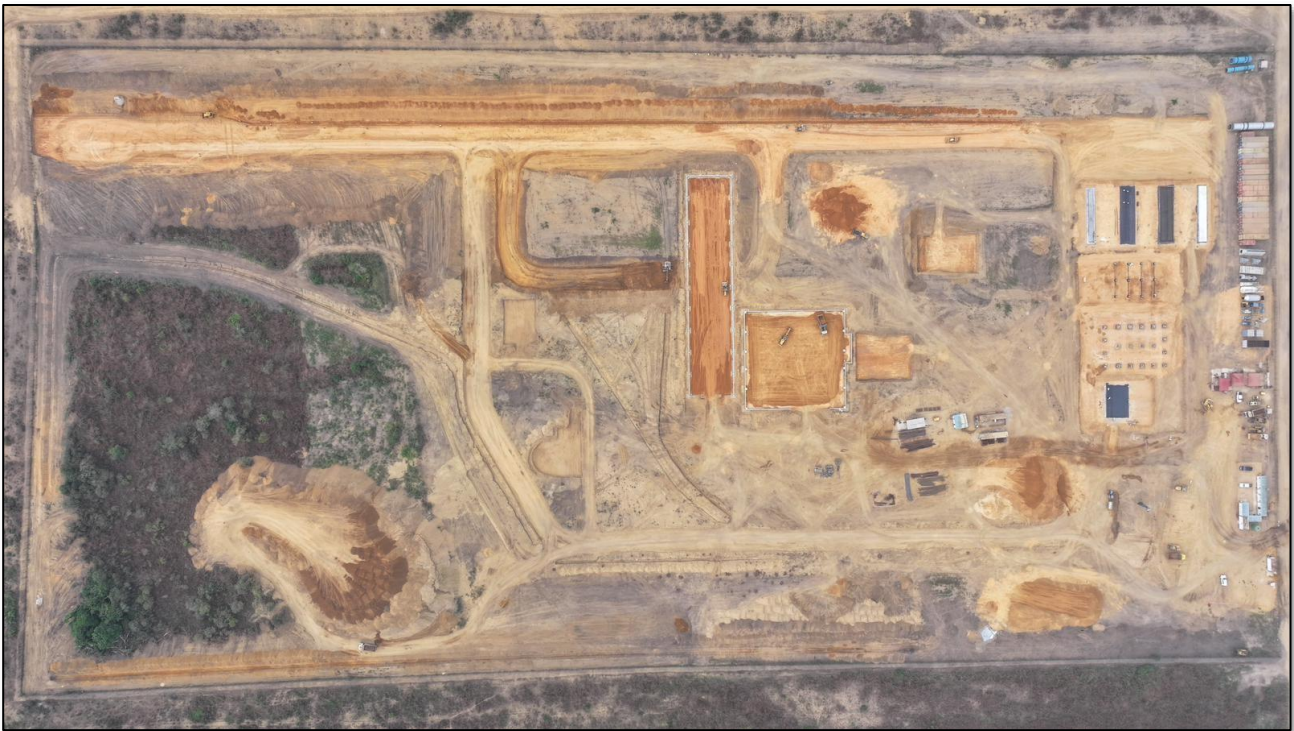
Figure 2 – Overall Progress at Company's Fertilizer Plant at 30 June, Subantando, Cabinda, Angola.
