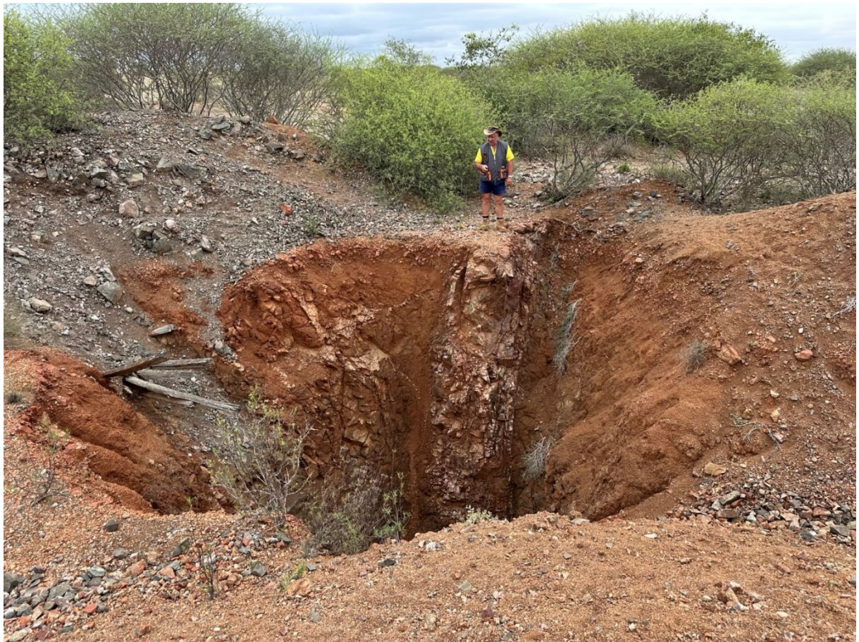
Figure 10: View west across the collapsed, main Cacimba shaft.
