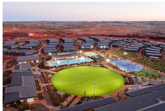
Mungala Resort at Ken's Bore completed
