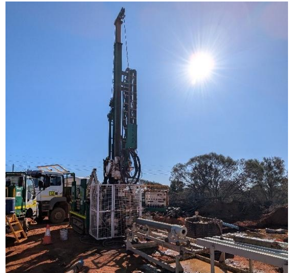
Figure 7: Large Diameter Drillholes core drilling is underway at the Goongarrie Hub.
