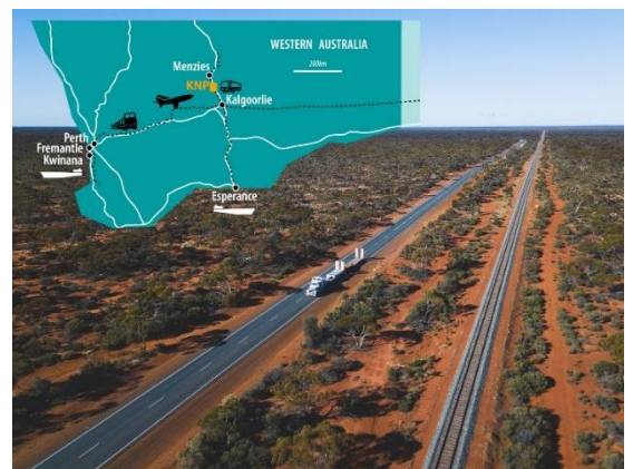
Figure 5: (below) Aerial image at Ardea's Goongarrie Hub at Goongarrie South, looking south towards Kalgoorlie-Boulder, showing road and rail infrastructure within the granted mining leases upon which the resources are located.
