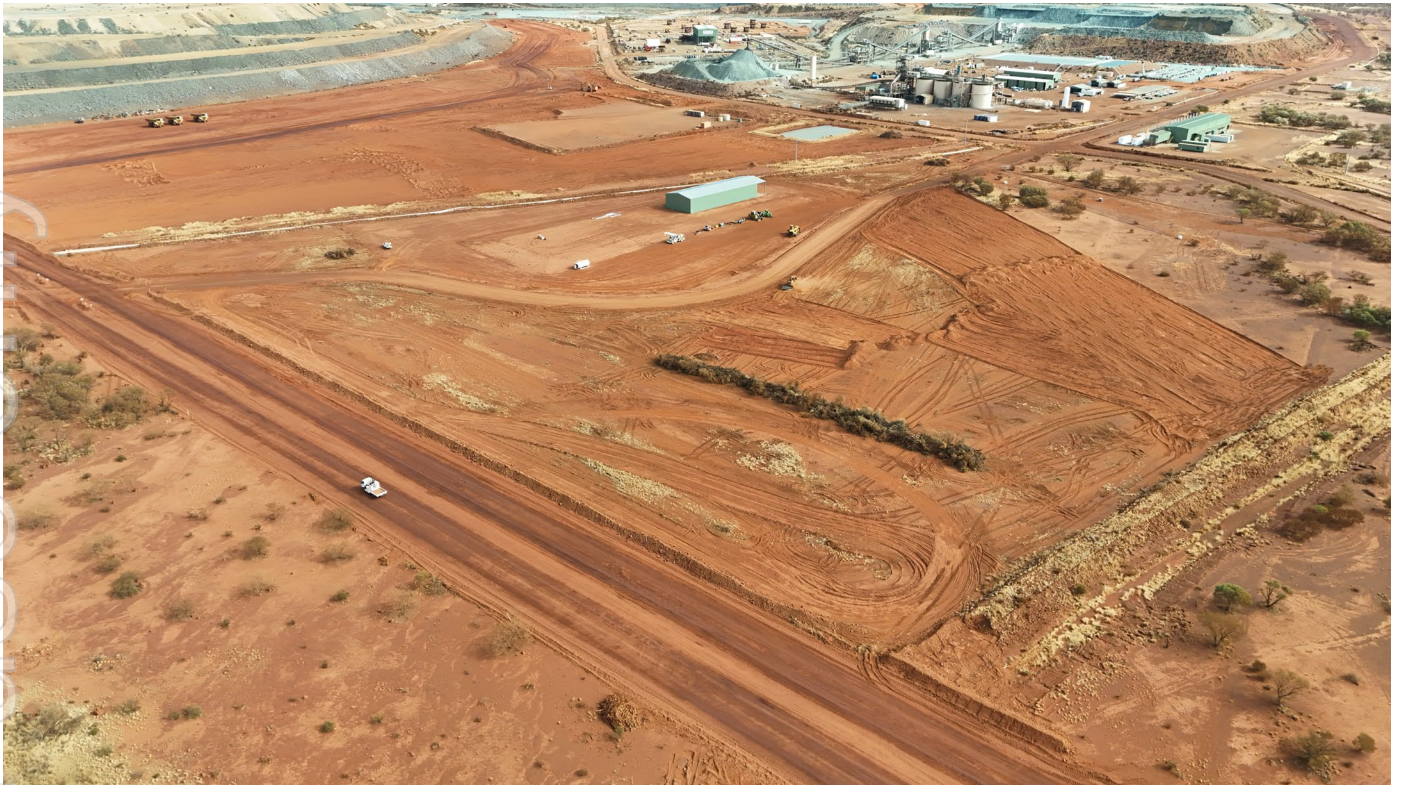
Karlawinda Expansion Project – Early Clearing Works
