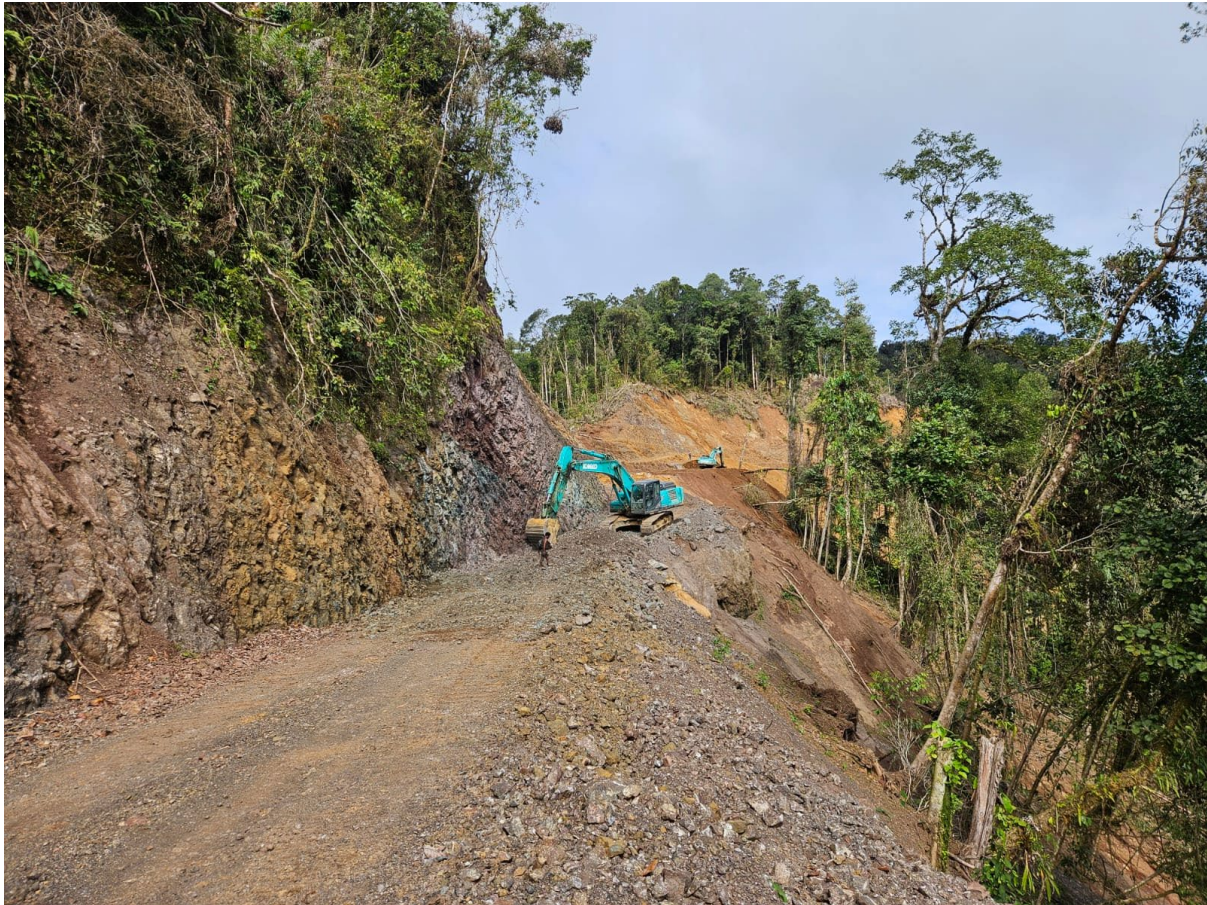
Photo 11: Tolukuma Access Road under Construction
