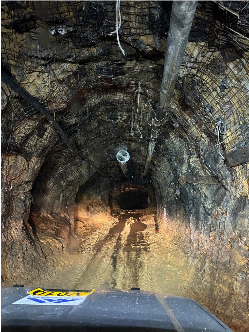
Photo 7: Good ground conditions and services installation in the 1565 portal
