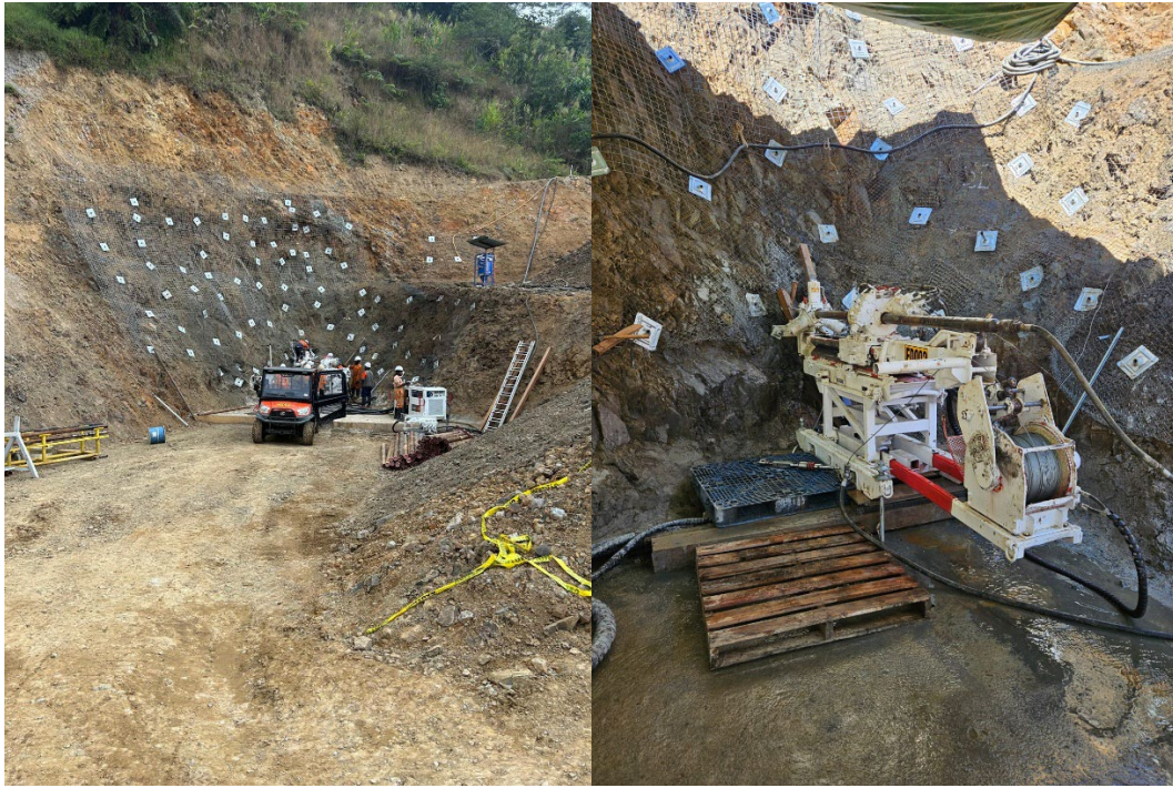
Photos 9 & 10: LM90 drill rig drilling the first dewatering hole, July 2025
