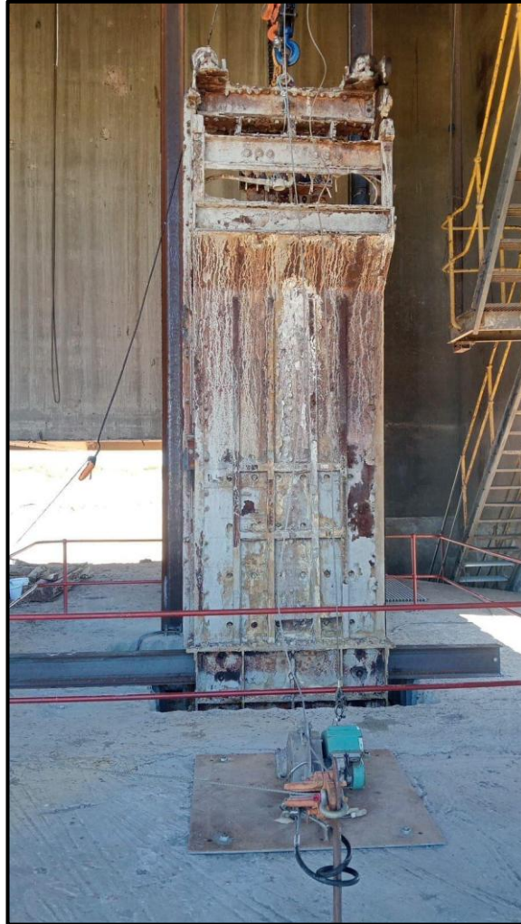
Photo 2: Hutchings Shaft cement slab opened and removed skip.
