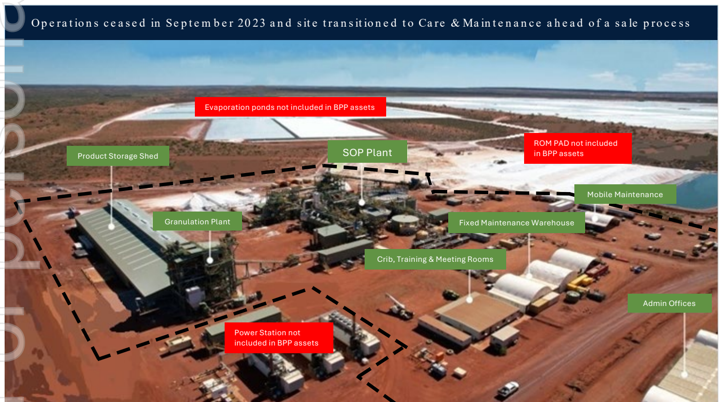
Figure 1 – Photograph of the Beyondie Potash Project in 2023 when in operation by Kalium. The Transaction comprises a fully constructed processing plant, site offices and maintenance infrastructure. Specific plant components include, KTMS crushing circuit, Kainite conversion circuit, column flotation circuit, liquor cooling heat exchangers, evaporative cooling circuit, product separation centrifuges, SOP recovery and granulation units, RO water plant and a bulk storage shed.
