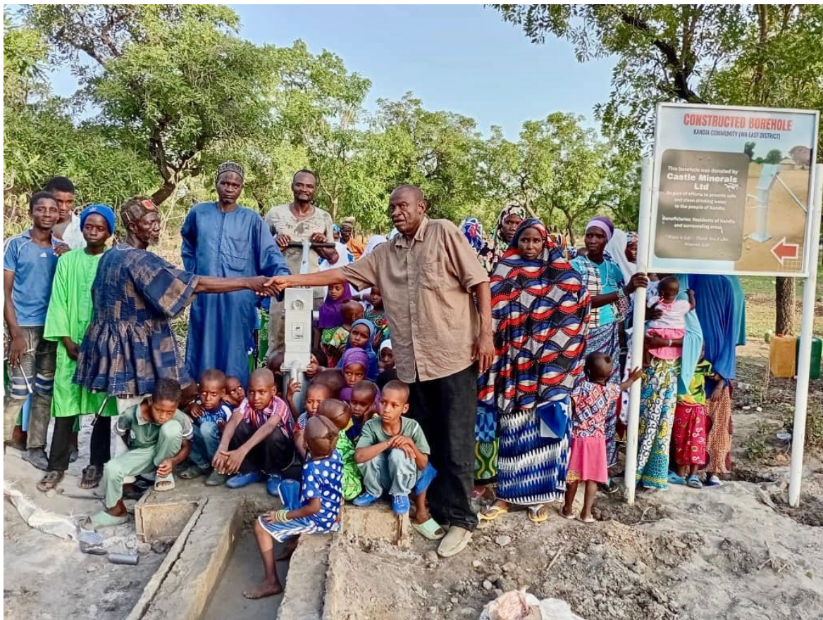
Fig 6: Castle's community manager, Ali Dauda, hands over a potable water borehole and pump to the Kandia community.
