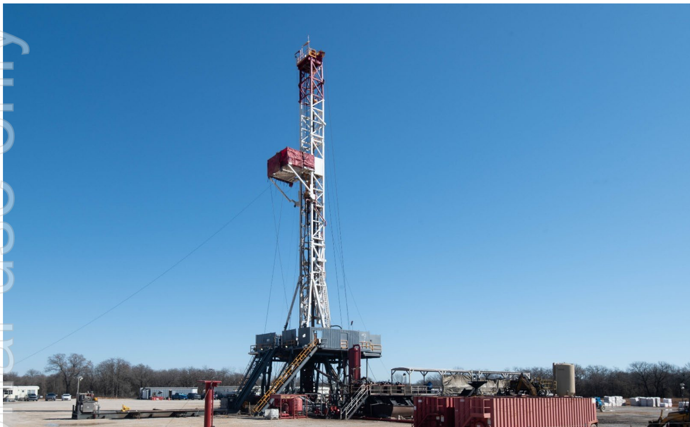
Figure 2. Bruins Well – Drilling Underway with Kenai Rig #19
