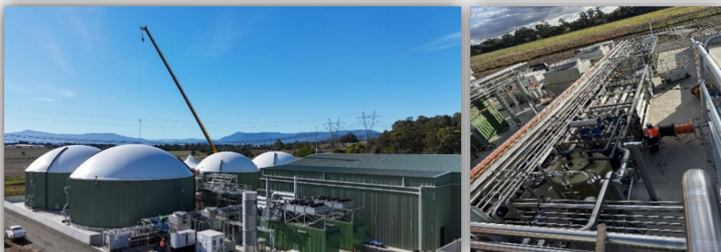
Image 3 & 4: YVW Bioenergy Plant construction
